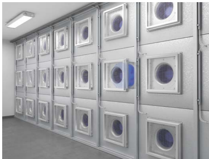
27 centrifugal fans with EC motors were installed on a wall construction as a multiple fan arrangement.
