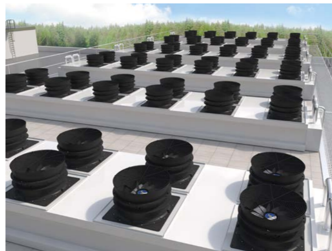
64 axial fans featuring AC technology were replaced with efficient ZPlus units.
