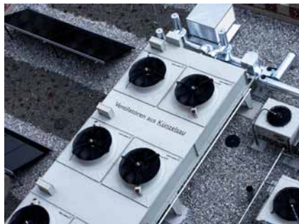
Condenser with axial fans
