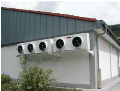
Small refrigeration units with ZIEHL-ABEGG fans
