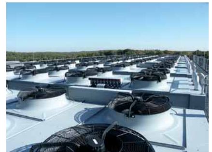
Condenser with axial fans
